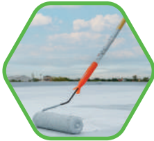
Waterproofing of terraces, sunken portion, chajjas
