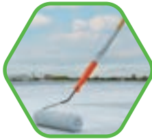
Waterproofing of terraces, sunken portion, chajjas, etc.
